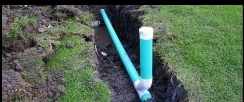
SEWER LATERAL CLEANOUT ALLOWS ACCESS TO LATERAL
